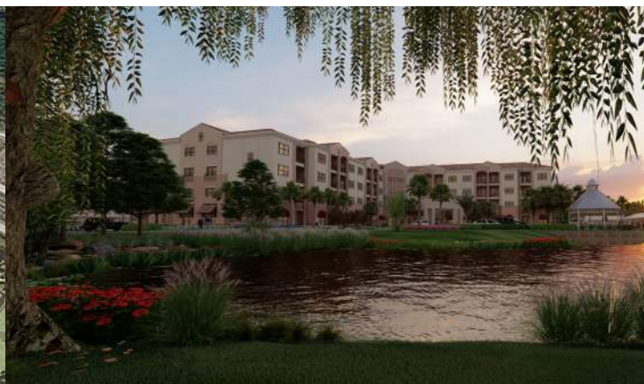
Assisted Living Facility, Florida
